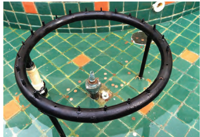
Figure 9. Fountain where the incident occurred. Note missing sprinkler head.
